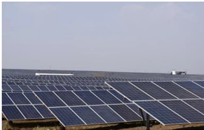
Solar park. Source: Vikram Solar GmbH. License: All rights reserved
